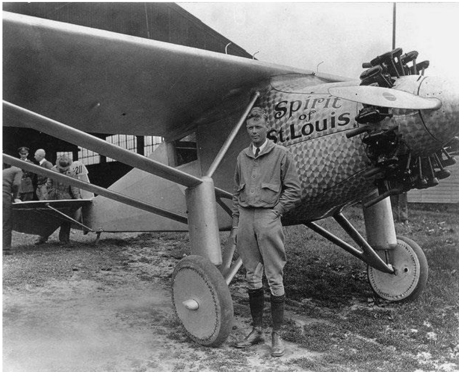
A confident-looking Charles Lindbergh standing in front of Ryan NYP, "The Spirit of St. Louis", a redesigned 1926 Ryan M-2 mail-plane powered by a 223 hp (166 kW) Wright Whirlwind J-5C radial engine. In order to make room for the extra fuel necessary for the cross-atlantic flight from New York to Paris and to maintain a stable centre of gravity, fuel tanks were built into what was formerly the pilot's and passengers' areas and the new pilot's compartment was located aft of them at the trailing edge of the wing. Special oil canisters were attached to the engine to keep it well-oiled during the flight.
