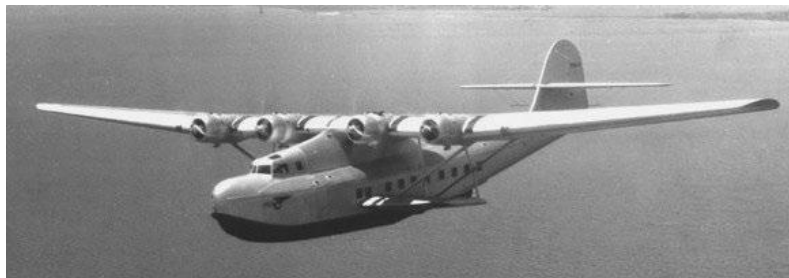
The streamlined and efficient early model Martin M-130 made the most of its total 3,800 hp whilst its competitors required 4,800 hp and more to perform the same task. Photo circa 1940
